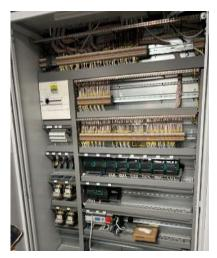
Fig. 2. The components related to data acquisition and network in the KTH live-in lab.
